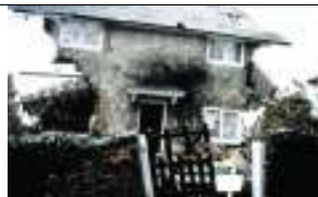
Impacts of landsliding & coastal erosion, Blackgang, Isle of Wight, UK
