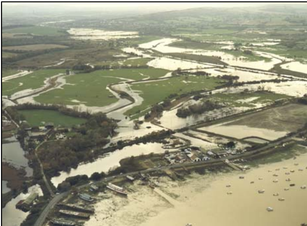
Bembridge Sea Wall (Embankment Road), part of the Strategy Area
